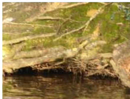
Erosion to the banks clearly visible.
